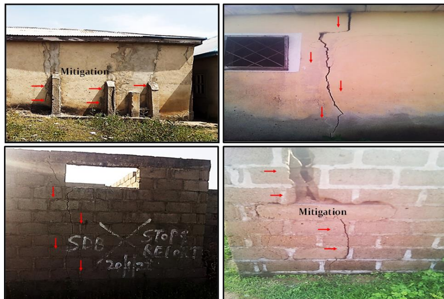
Figure 1: Mitigation measures on cracked building
